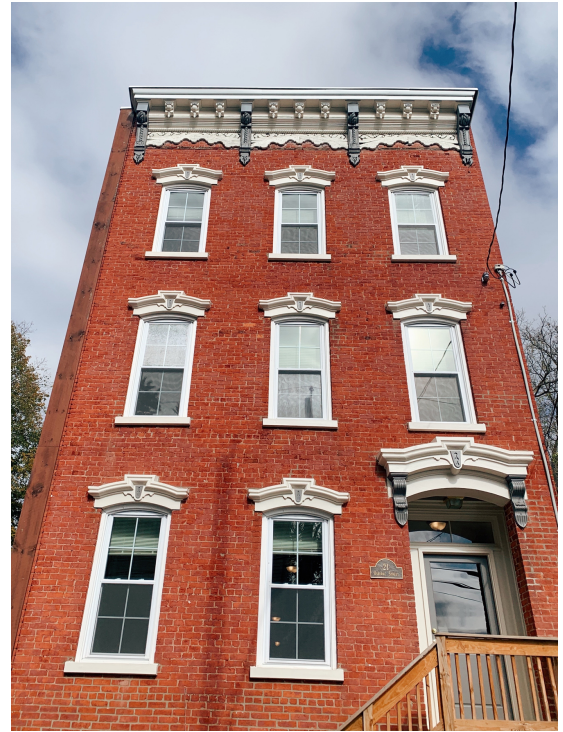
Fully rehabbed, two-family Habitat home in Albany's South End
